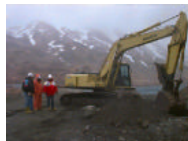
Inspecting berm fill
