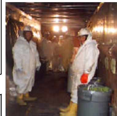
Workers in decon area
